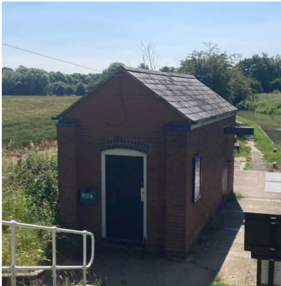
Plate 3-3: Example of existing pumping station
